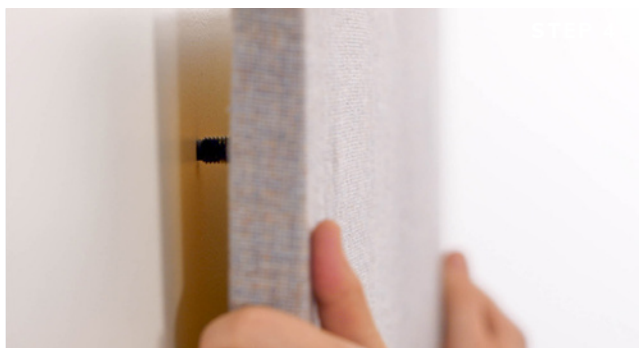
Push the panel onto the black ratchets to make indentations in the panel core material.
